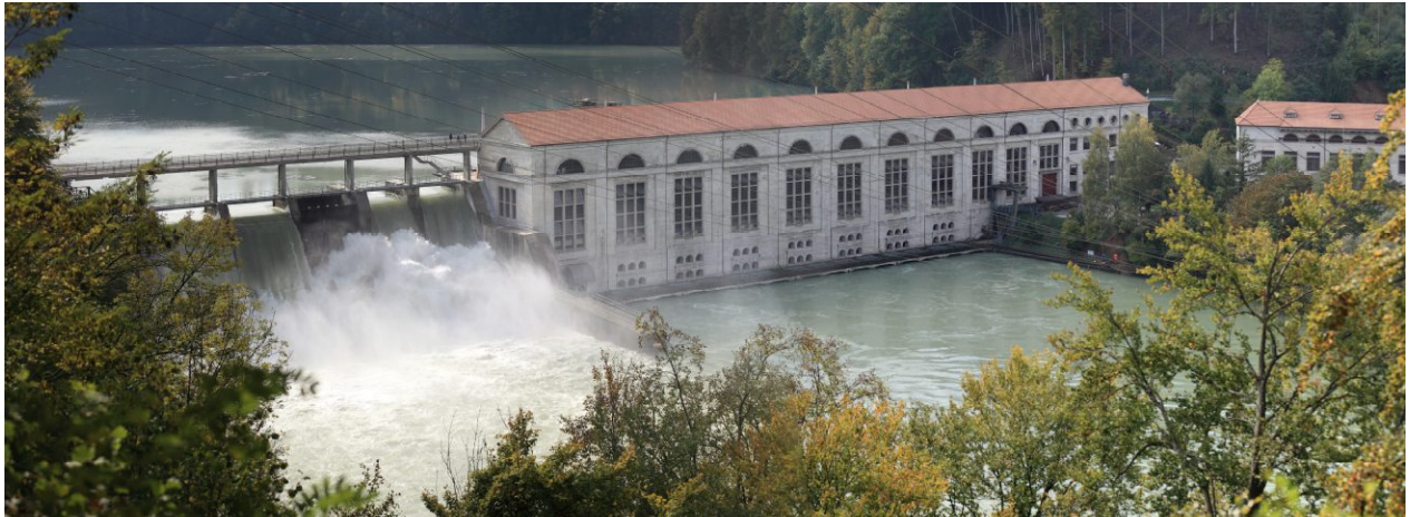
Fig. 8 Mühleberg dam (1920, 19 million m 3 ), 1.2km upstream of KKM performing flood waters release during the surprising 2011-10-10 “rain on snow” event that caused great damage in the Bernese Alps 16 .
