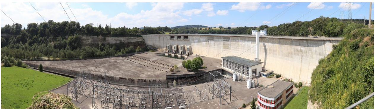
Fig. 10 Schiffenen dam (1963, 58.6 million m 3 ) on river Saane. Recent evaluation shows 17 , that the flood from the Rossens failure will overtop the Schiffenen dam by 8m. Photo/panoramic: M. Kühni, 2011
